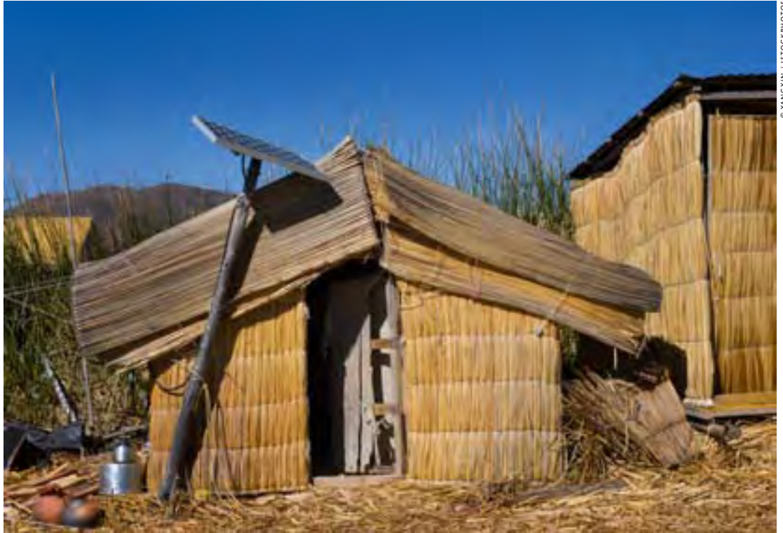
Solar panel at hut on Lake Titicaca in Bolivia
